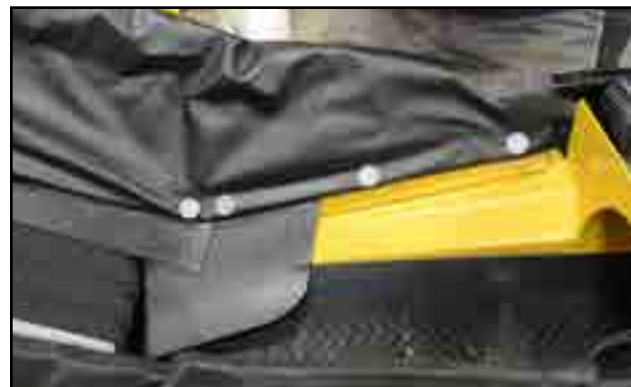
Fig 104 - Transition corner flashing in place
