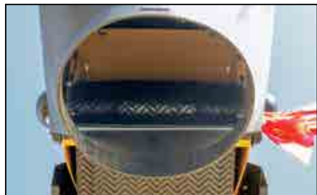
Fig 83 - Inside discharge spout
