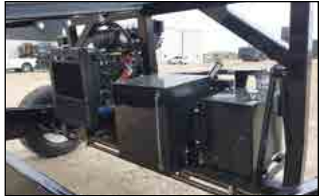
Fig 12 - 22110 fuel tank and hydraulic reservoir
