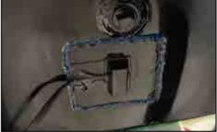
Fig 28 - Oil reservoir heater
