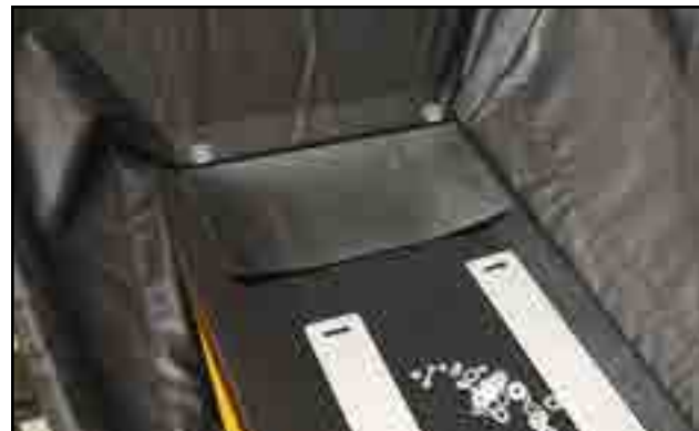
Fig 103 - Tail flashing on top of side flashing
