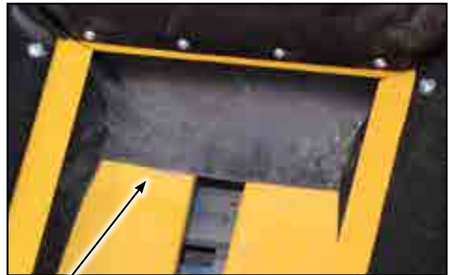
Fig 99 - New tail flashing
